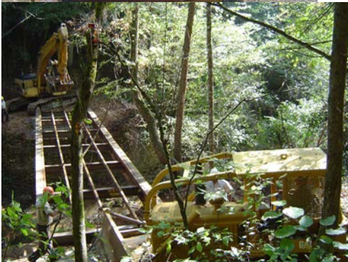
Bridge steel frame is set in place
