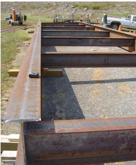
Bridge steel frame components delivered to W. Kerr Stott Dam for assembly
