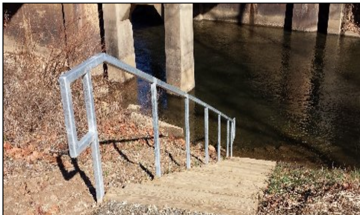
Steps located below the Hwy 421 Business Bridge along the Reddies.
