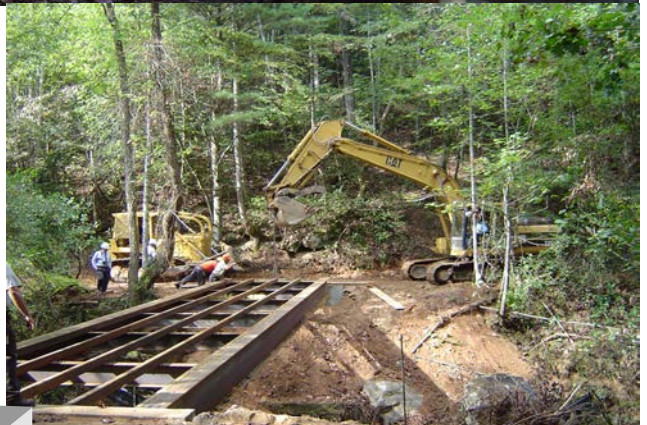
Bridge steel frame is set in place
