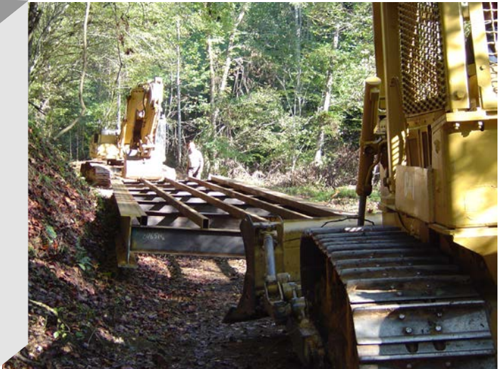
Bridge steel frame components delivered to W. Kerr Stott Dam for assembly
