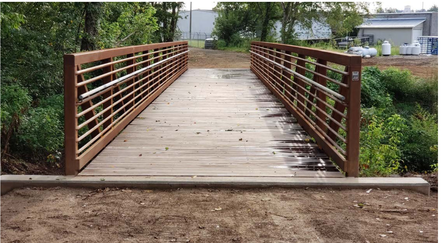
Memorial Park to Mulberry Fields Connector bridge completion!!!!
